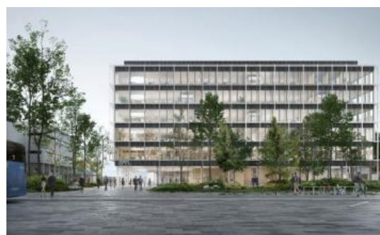
ASB - Advanced Science Building - EPFL Lausanne
